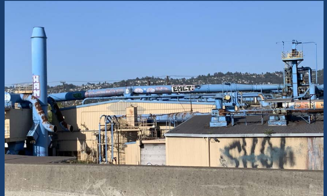
Photo: View of the former Pacific Steel site from I-80
